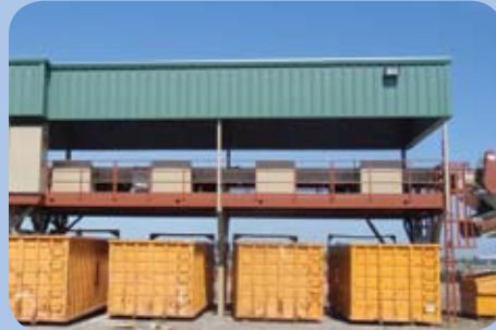
RCTS's new Construction and Demolition Recycling Program.
